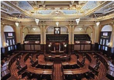
The Illinois House Chambers with faux wood-finished steerable line array speakers flanking the white center columns, voting/video displays on the side of the room, and custom 34-inch gooseneck mics folded into historically accurate, reconstructed legislator desks.
